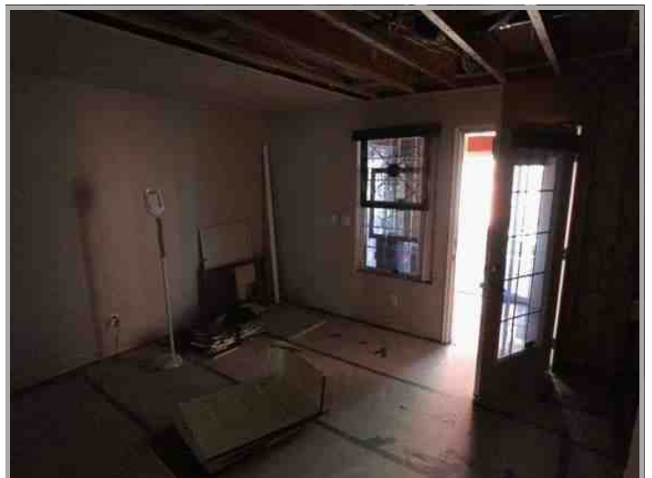
Basement Den/being repaired
