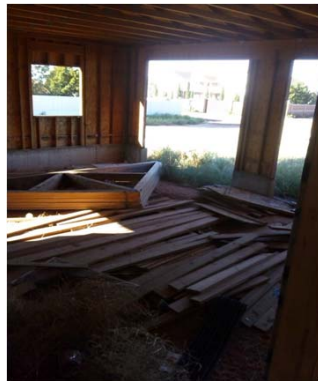
Dirt floor in Garage
