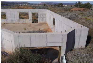
Concrete Slab and Walls
