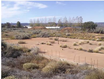
Pipes exposed to the weather
