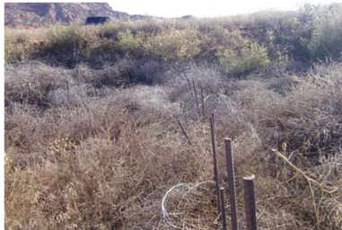
Reinforcing for entry slab
