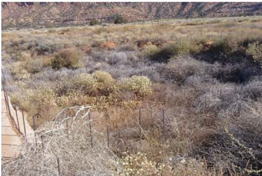
Footings for entry
