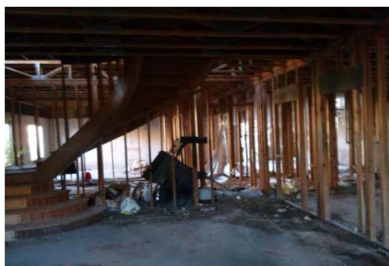
Interior view at basement
